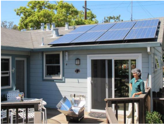
Courtesy Sunwork Renewable Energy Projects
